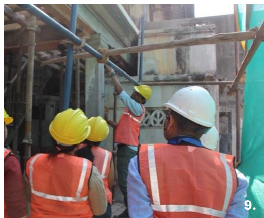
Image 9: Assessment of the out of plumb wooden column at the front wing of the house with Mehul Shah
