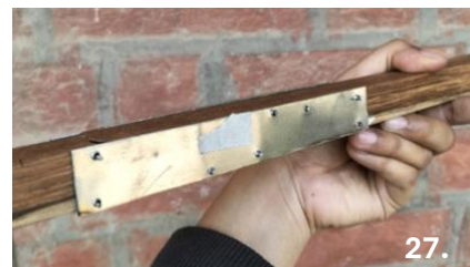
Image 23: Nigar Shaikh explaining the various methods to repair damages in timber structures through models. Image 24,25,26,27: Examples of various joineries used to repair a timber beam.
