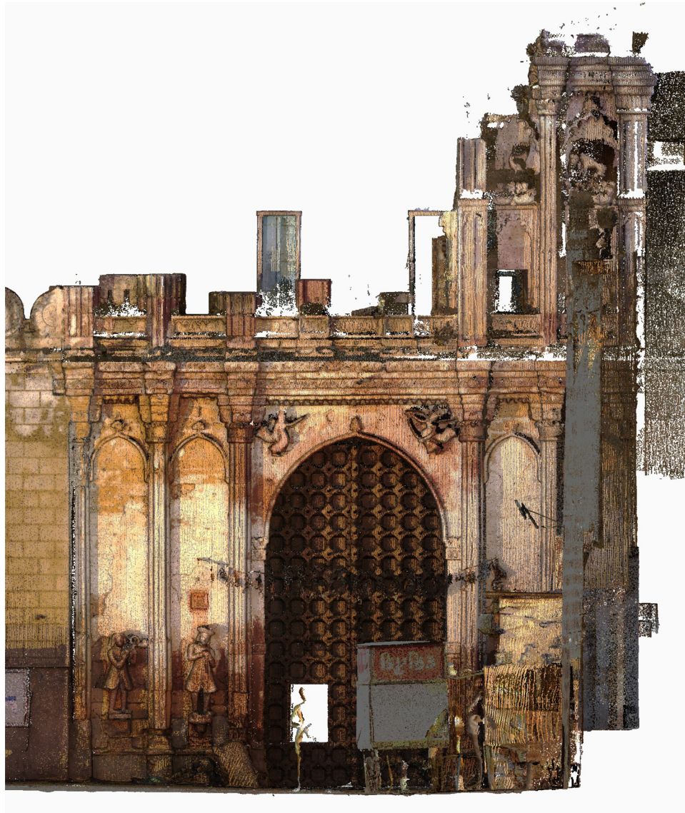
Elevation view generated from the 3D point cloud model of Nagarkhana, Darbargadh, Kutch by V. Purohit as part of MCR 2021, CEPT University. Data collected by workshop participants under the guidance of M. Mane, Z. Pithawalla, D. Nakrani. Post processing and Visualization by M. Mane, Z. Pithawalla, and D. Nakrani for CHC - CRDF.
