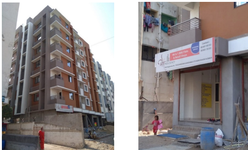
Figure 26: Images showing (L) the project (R) a shop in Om Residency, Vastral Source: Compiled by authors
