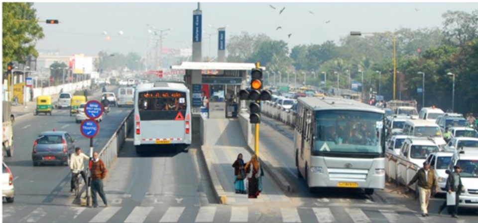
Ahmedabad BRTS creating an example for Queue jumper Source : Planning, design and development of BRT by CRDF
