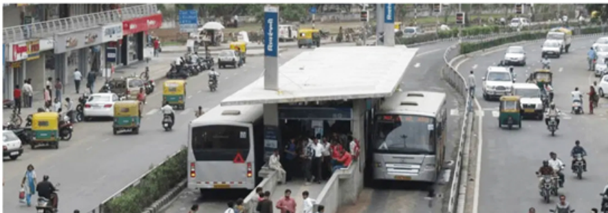
Single Median Bus Stop (Ahmedabad BRTS) Source: Planning, design and development of BRT by CRDF
